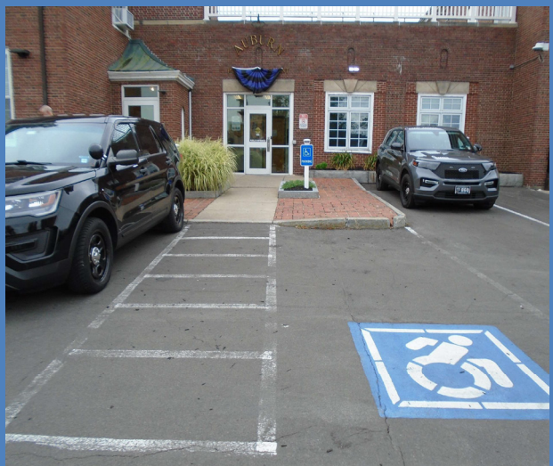
No van accessible parking, accessible aisle too narrow and sign is too low at the Police Station.
