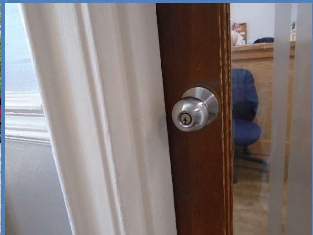
Office doors at the Town Hall have doorknobs, and not accessible handles such as latches or levers that can be operated without grasping or twisting.
