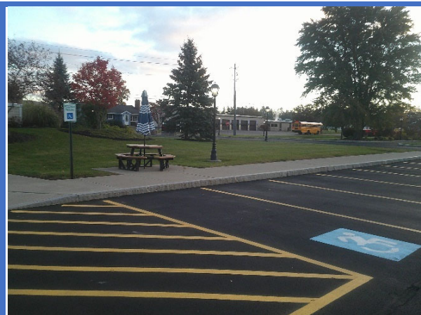
None of the accessible parking spaces at the Town Hall have a sign indicating they are van accessible.
