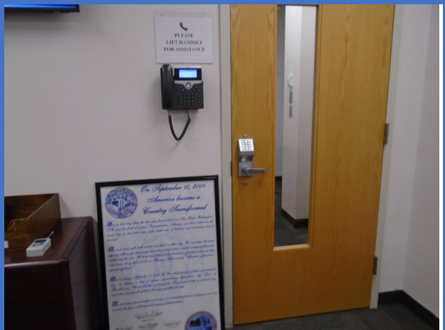
Intercom at the Town Supervisor's Office mounted higher than 48 inches; potentially inaccessible from a wheelchair.
