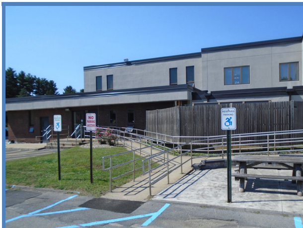
No "van accessible" signs at van accessible spaces at the Town Hall.
