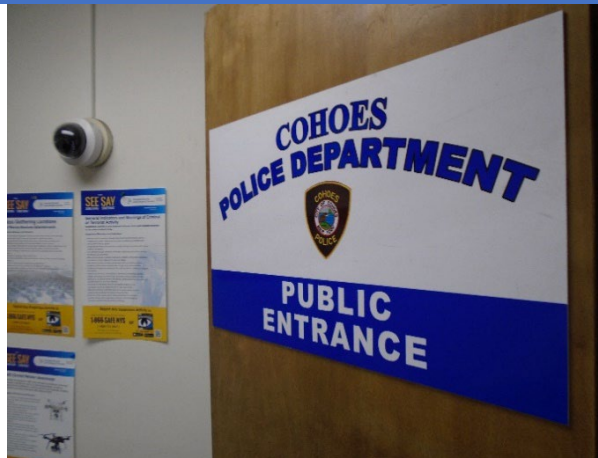
Police Station entrance sign lacking raised lettering and Braille.
