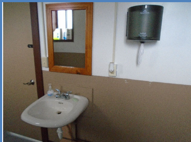
Restroom hand towel dispenser, mirror and door lock are mounted too high.
