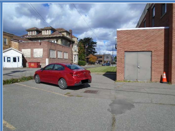
No accessible parking spaces in public parking lot at the Police Station.
