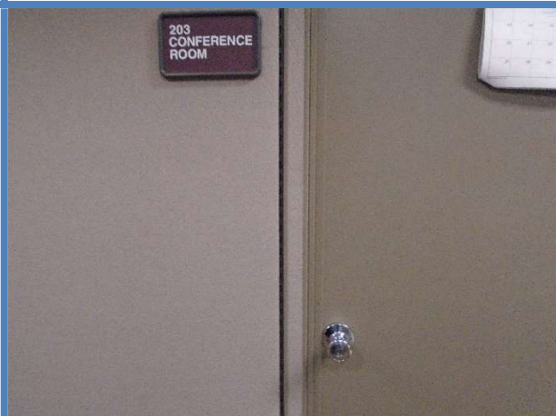
Conference room door has doorknob, and not an accessible handle such as a latch or lever that can be operated without grasping or twisting.
