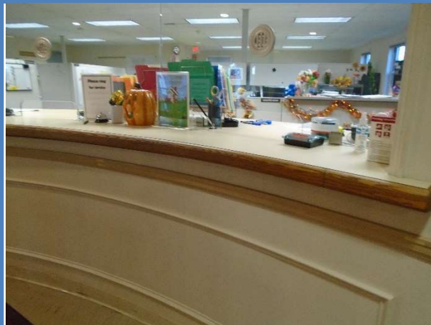
Service counter in the Town Hall without an accessible portion no higher than 36 inches.
