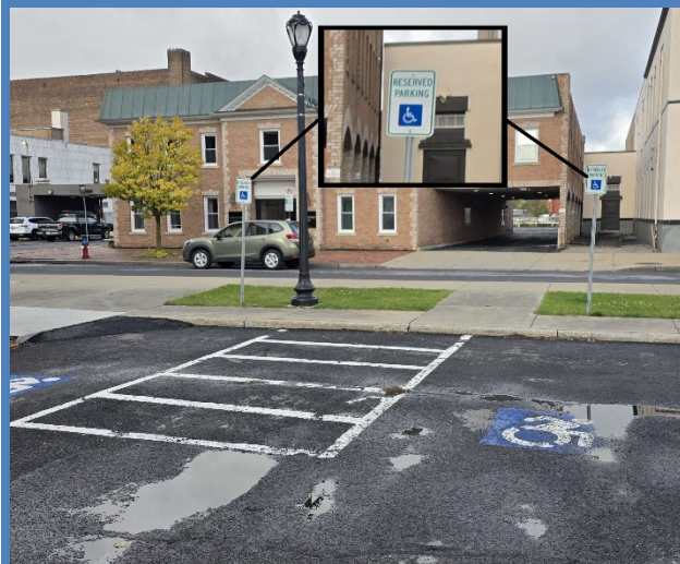
No signs identifying van accessible parking spaces at City Hall.
